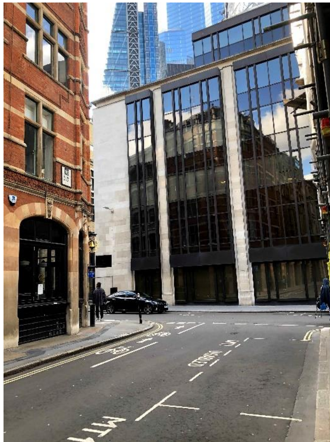
Figure 2:View of Bury House from Mitre Street
